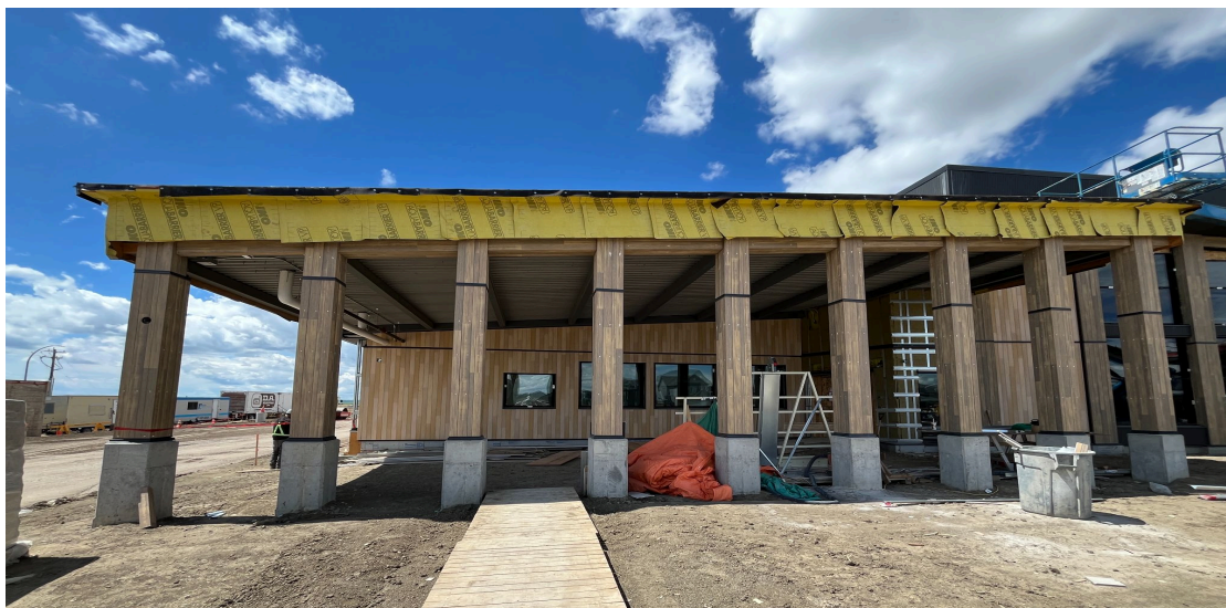
Below: Front Entrance Canopy
