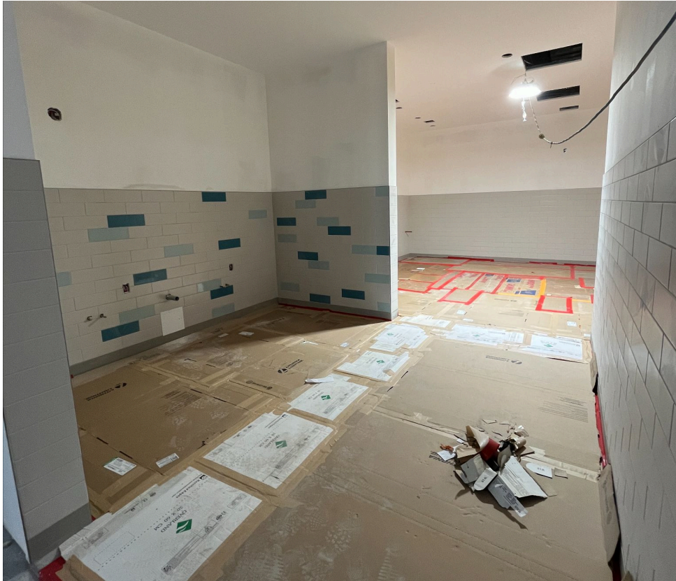
Above: Tiled Washroom
