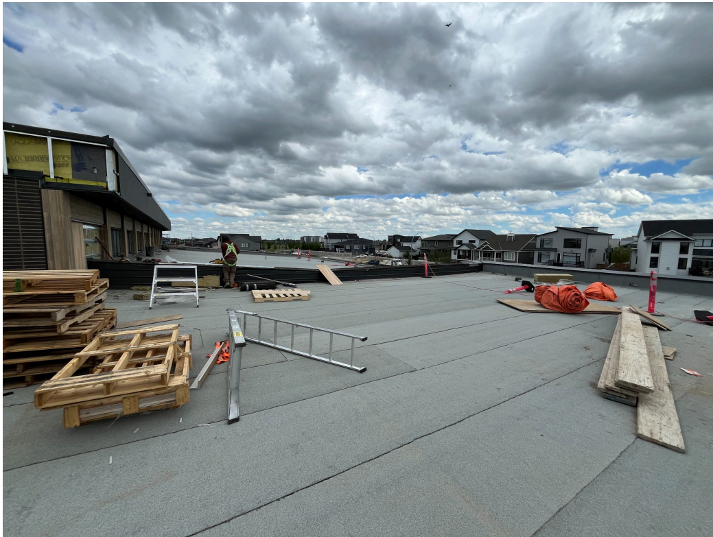
Above: Roof View Looking Southeast
