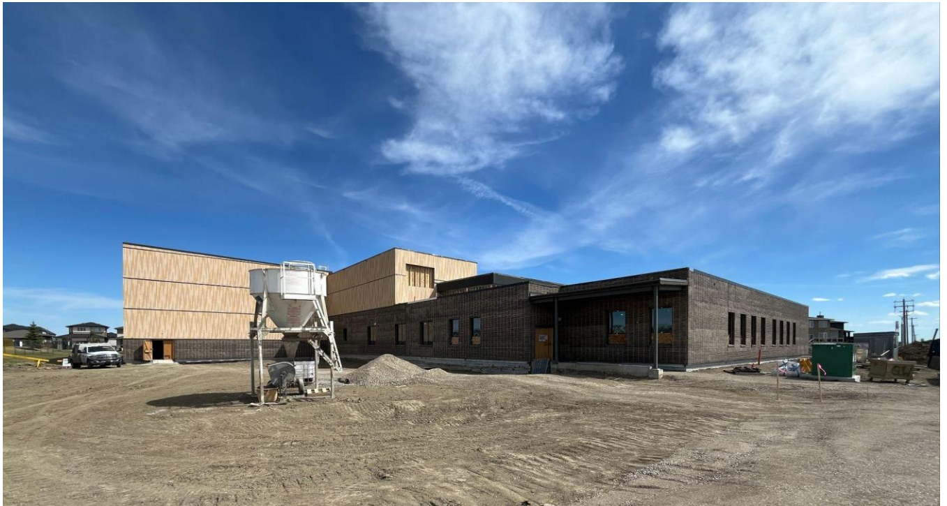
Below: Northwest Face
