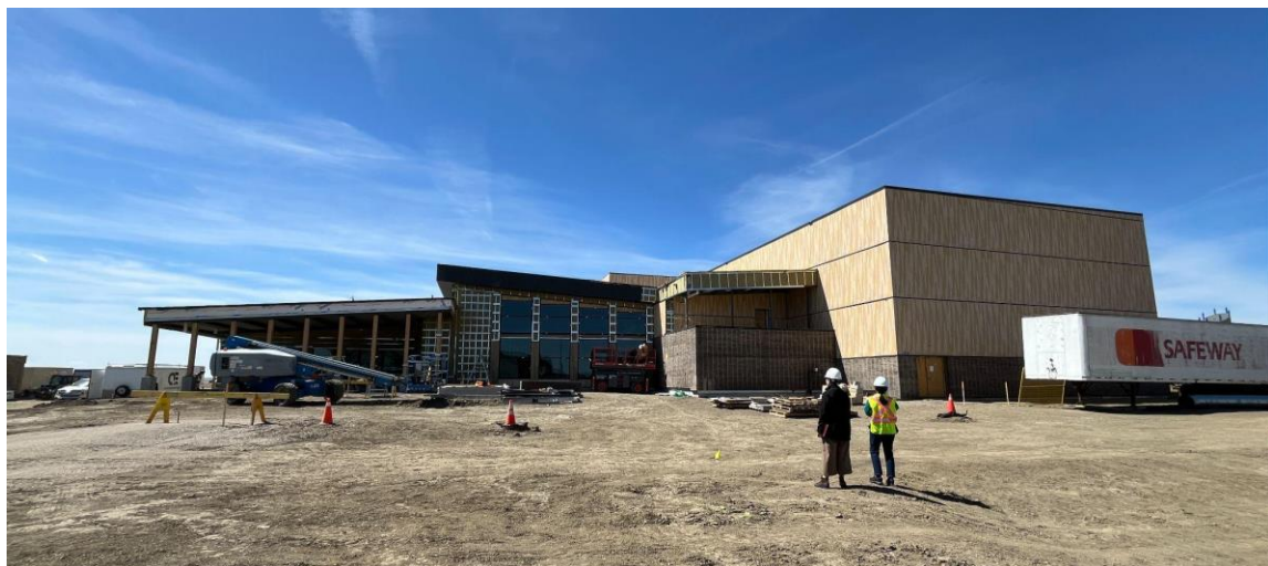
Below: East Face
