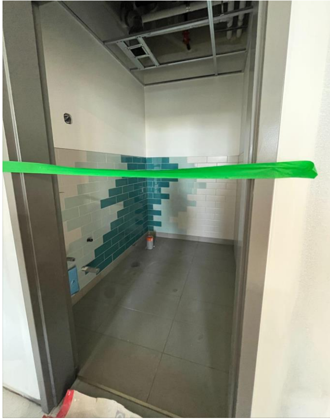
Above: Kindergarten Washroom Tilework
